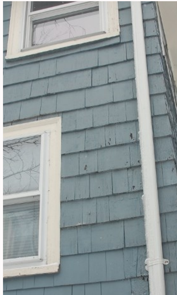
New round downspout painted the same color as the house trim.
